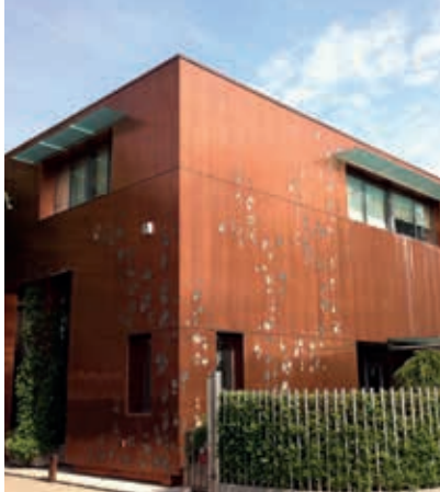
COPPER PANELS - ITALY
