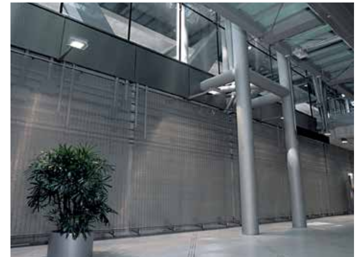
Cladding of technical systems Terminal 2, Cologne-Bonn Airport, Germany.
