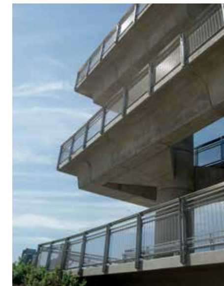
Semi-transparent balustrade infill Malcom Martin Platform, St. Louis, USA.
