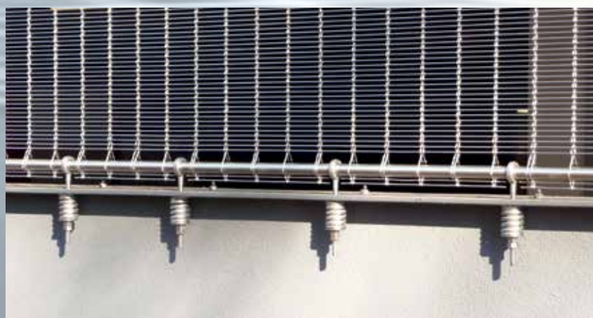
Bottom mounting: round bar with eyebolts and pressure springs.
