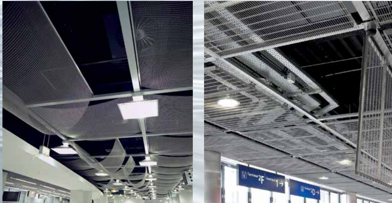
Adjustable mounting system for ceilings with sag.
