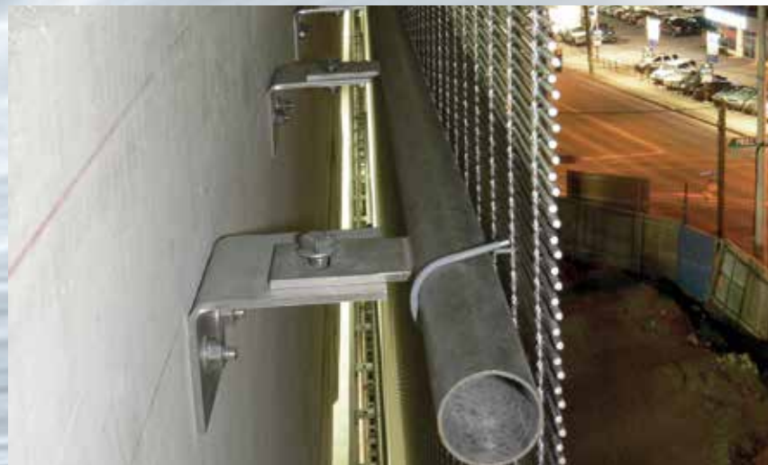
Intermediate mounting: round tube and wire connectors.
