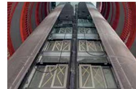
Lift shaft cladding with architectural mesh, Ulm Town Library, Germany.
