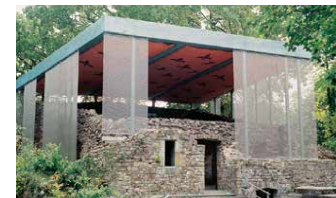
A semi-transparent stainless-steel mesh encloses the existing building and ensures natural lighting. C&A Eco Store, Mainz, Germany.
