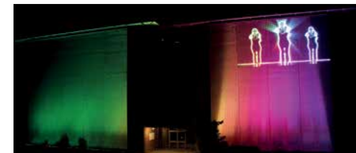
Mesh illumination. Haver & Boecker office building, Oelde, Germany.
