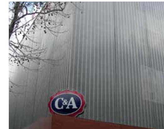
A semi-transparent stainless-steel mesh encloses the existing building and ensures natural lighting. C&A Eco Store, Mainz, Germany.
