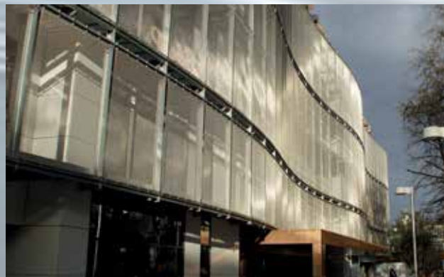
Wave-shaped façade cladding: Holland Park School, London, Great Britain.
