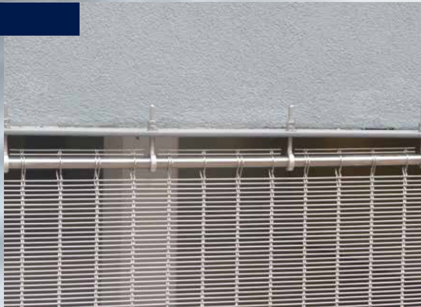
Top mounting: round bar with eyebolts.
