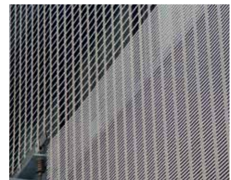
The precisely defined open area breaks up and filters sunlight creating a pleasantly cool and bright interior climate.
