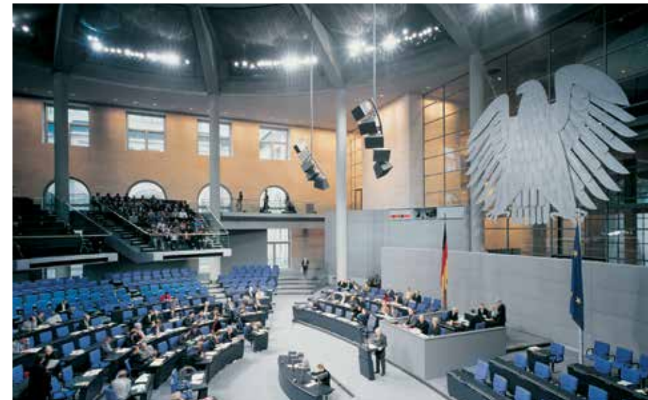
Modern acoustic fleece behind an elegant stainless-steel veil. Plenary Hall of the Reichstag building, Berlin, Germany.
