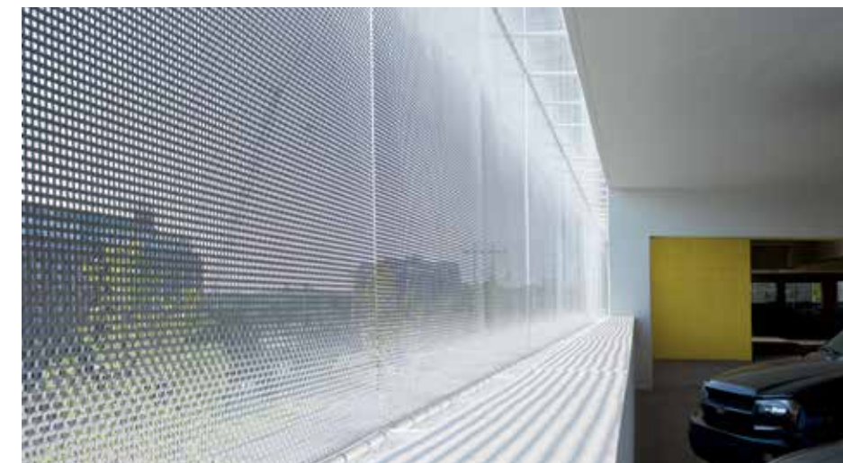
Sun protection with a good view from inside. Multi-storey car park, Chesapeake, Oklahoma, USA.
