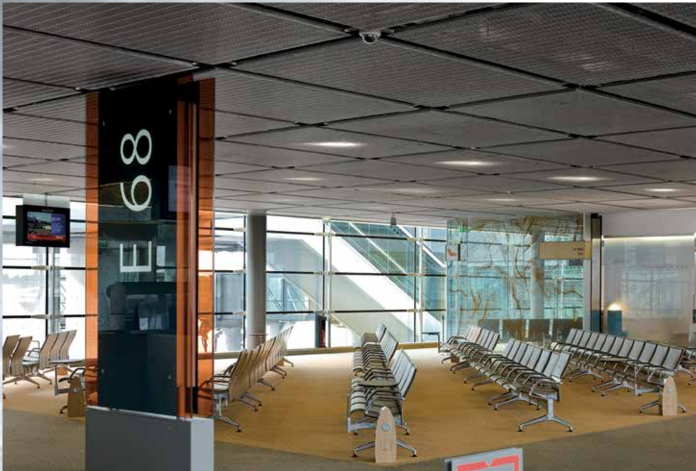
Architectural wire mesh guarantees the optimum operation of ventilation or sprinkler systems Terminal S3, Roissy Charles de Gaulle Airport, Paris, France.
