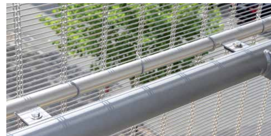
Intermediate mounting: round tube and wire connectors.
