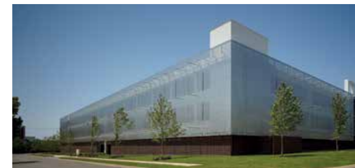
View during the day. LARGO-PLONUS wire mesh, Car Park Chesapeake, Oklahoma, USA.
