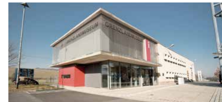
EGLA-TWIN wire mesh façade during the day. Eichsfeld Borderland Museum, Teistungen, Germany.
