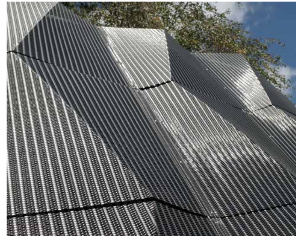
3D mesh façade by Haver & Boecker for mesh cladding with a dynamic effect.
