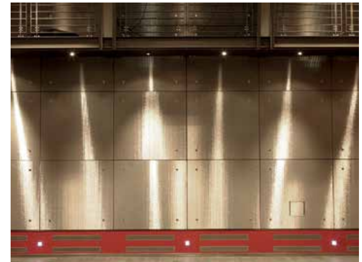
Architectural mesh makes the walls of the proscenium at Luxembourg's Théâtre Municipal shine.
