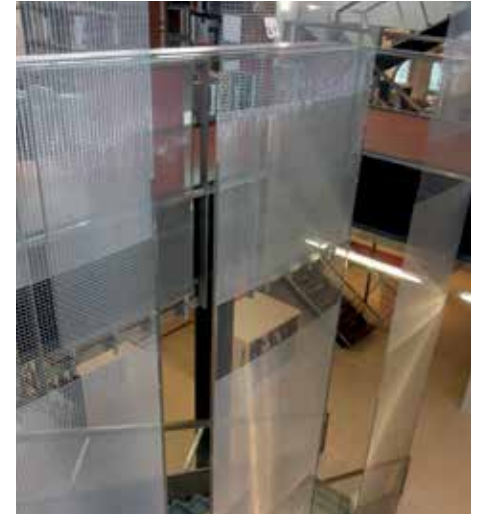
Mesh with varying aperture widths. Mediathèque Chateaugiron, France.
